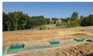
INSTALLATION FOSSE SEPTIQUE
